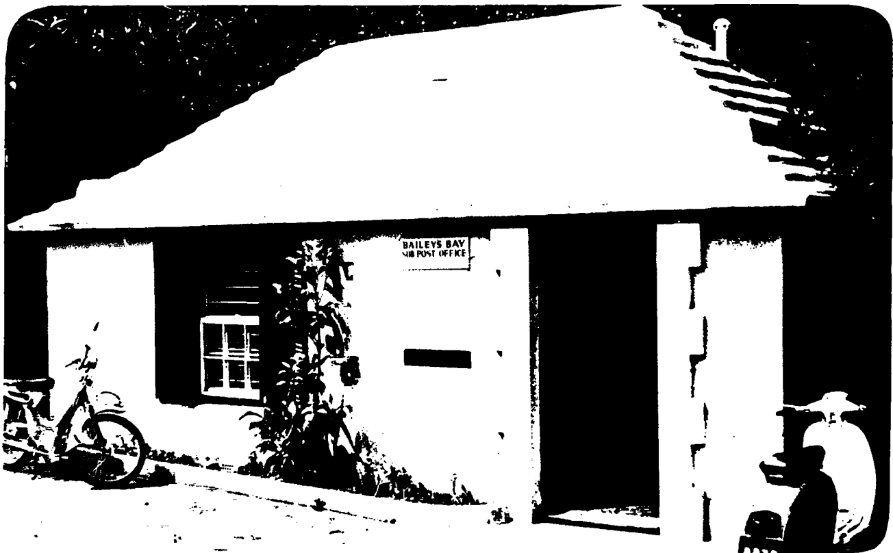
BERMUDA'S SMALLEST POST OFFICE BUILDING IS THAT AT BAILEY'S BAY. ORIGINALLY BUILT AS THE LOCAL JAIL, IT NEVER SERVED AS SUCH. Photo by Dr. J.C. Arnell
