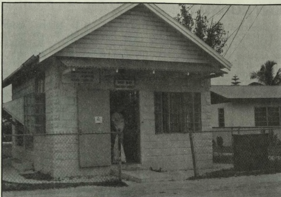
Fig. 10 West Bay Sub-Post Office
