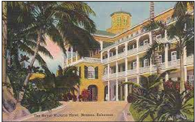
Figure 4 An exterior view of the front of the Royal Victoria Hotel in Nassau, Bahamas.
