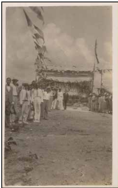
1043 Entrance to North Side, opening new road, 1935.
