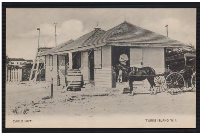
Fig. 1 Cable Hut Turks Island
